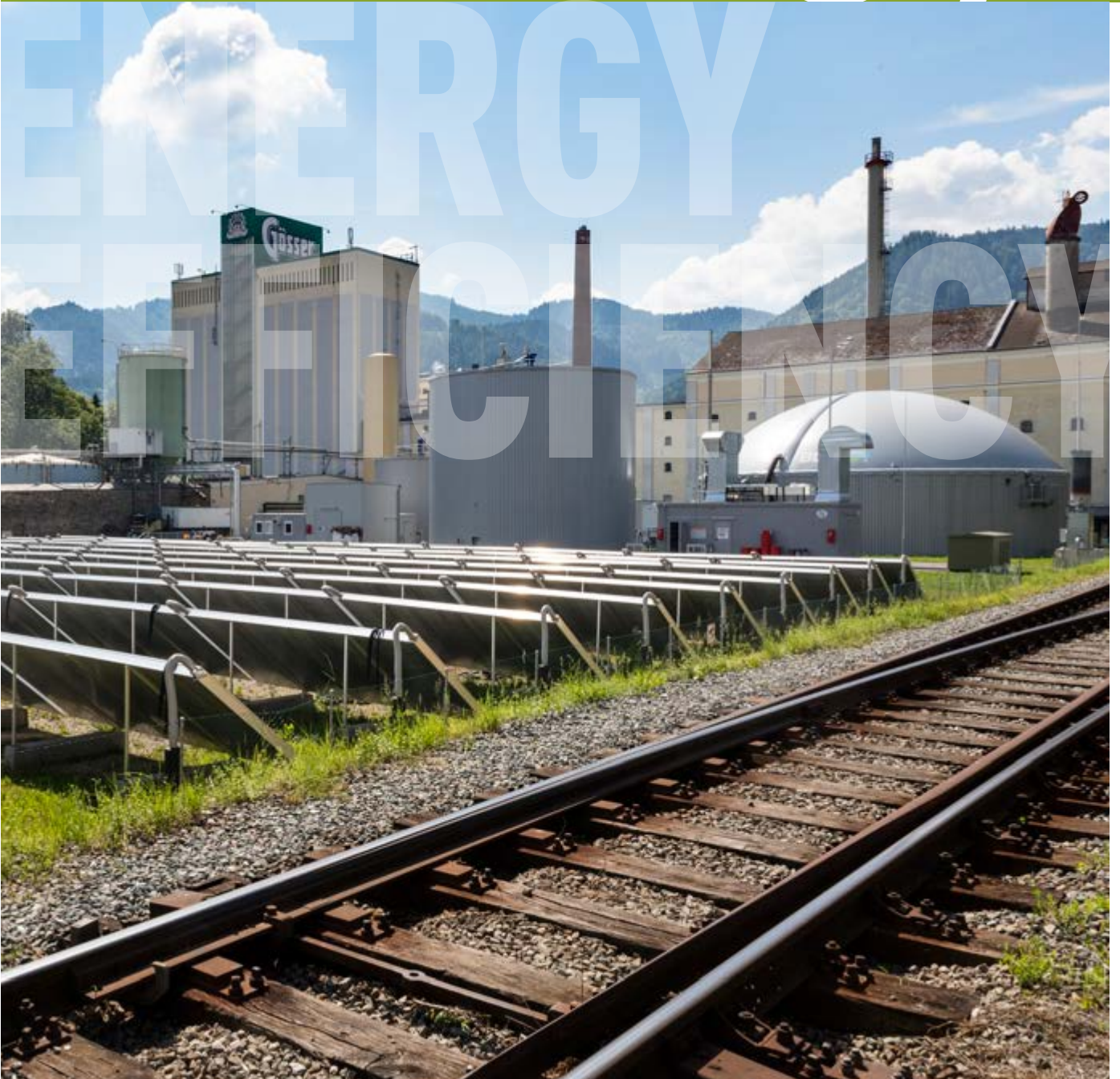
Solar thermal plant (bottom left) and a spent grain fermentation tank for biogas (centre) at Göss brewery of HEINEKEN in Leoben, Austria.
